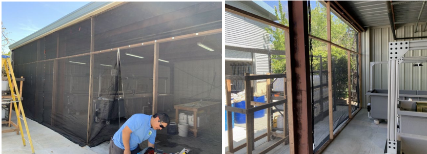
Figure 2 Image of the constructed screened in-wall to the Fish Hatchery.
