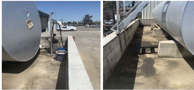
Figure 4B Image of the oil tank area after it was cleaned and decluttered.
