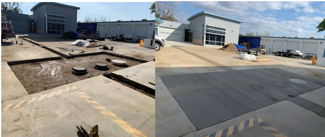
Figure 6. Before and after images of the District plumbing project.
