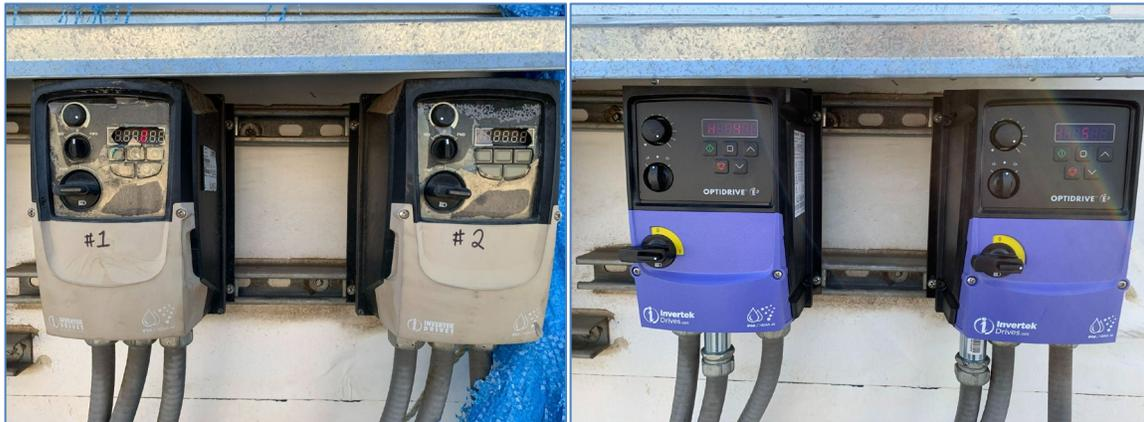
**Figure 7.** Old VF drives (left) and their replacements (right).
