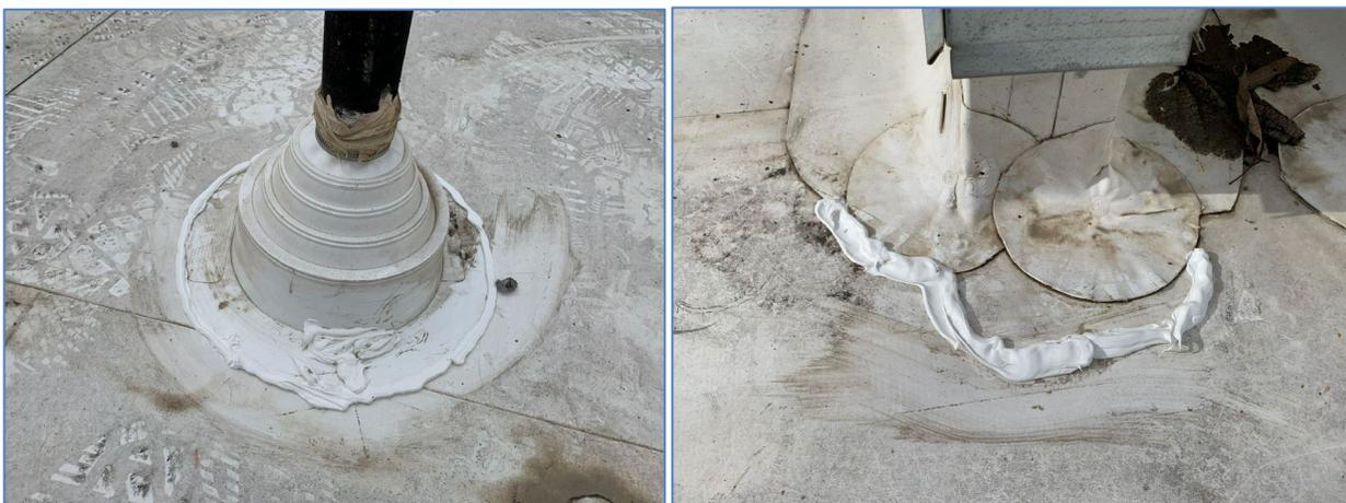
**Figure 6.** Temporary repairs to prevent water leaks on the roof of the fish hatchery. The TPO boot (left) was repaired and the patch seals (right) checked.
