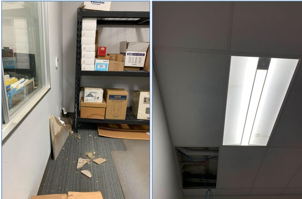
**Figure 5.** A water leak caused minor damage to the offices in the new fish hatchery building.
