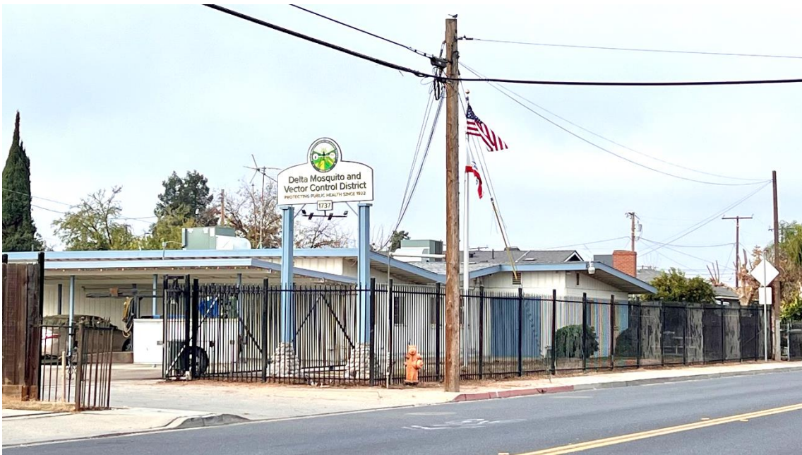
Figure 1b. View of the new fence
