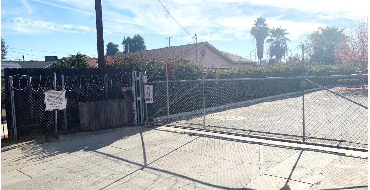
Figure 2a. View of the old rolling gate.
