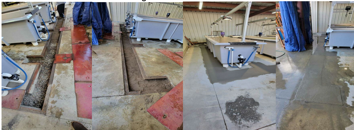
Figure 7. Before and after images of the repaired floor around the outdoor fish tank area.
