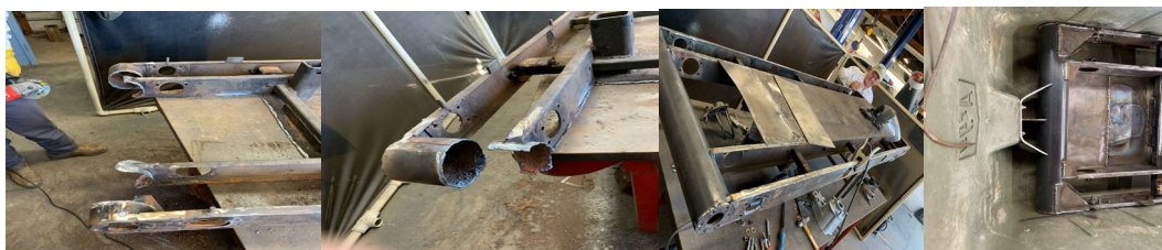
Figure 4. Image of the replacement of T-29 Argo's damaged frame with a new metal frame
